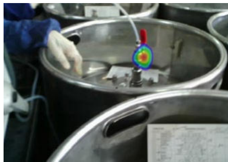
Gas pipeline leakage
